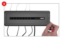
Once you are sure that all wires are correctly connected, install the top cover and connect the wiring centre to the 230 V power supply – the red "Power" LED will light up.
